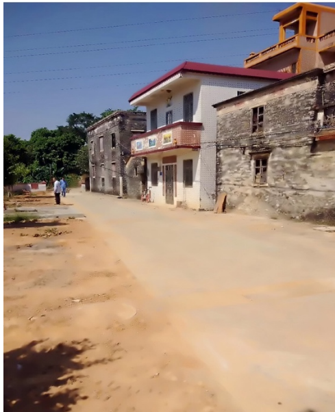
Town Hall (with balcony)
